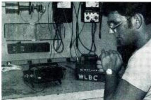
WLBC engineer Steve Brown uses a counter to measure the frequency of a portable transceiver on the bench. While the readouts did not show up in the photo, they usually are easy to read at some distance.
